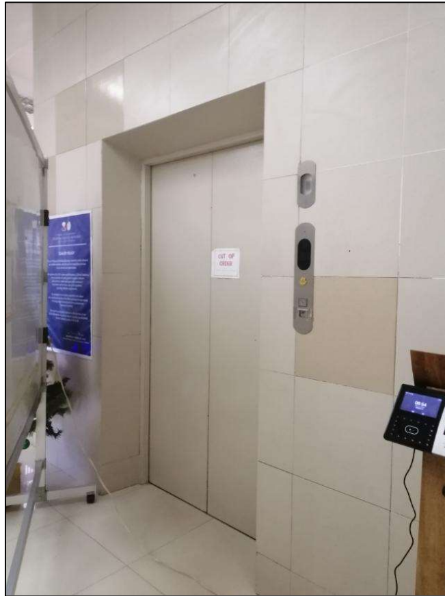
Dismantling/Decommissioning of Existing Elevator
