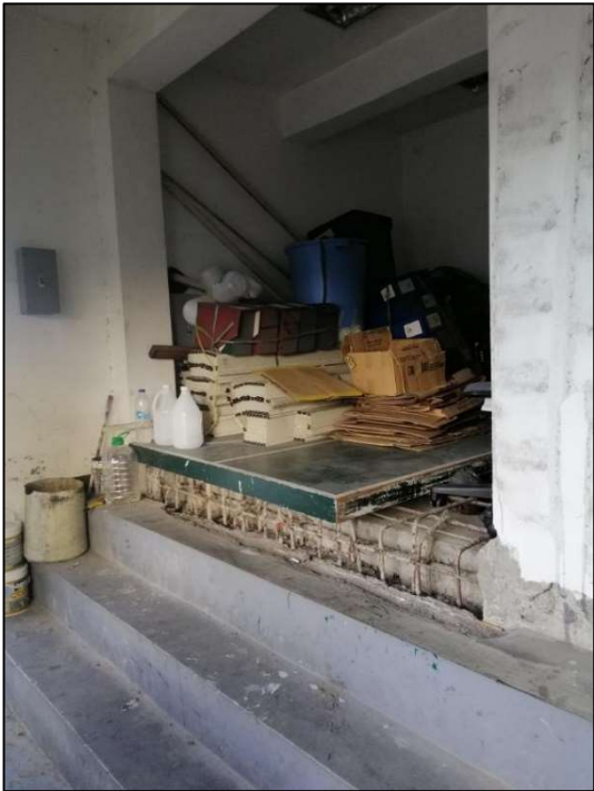
Elevator Machine Room
