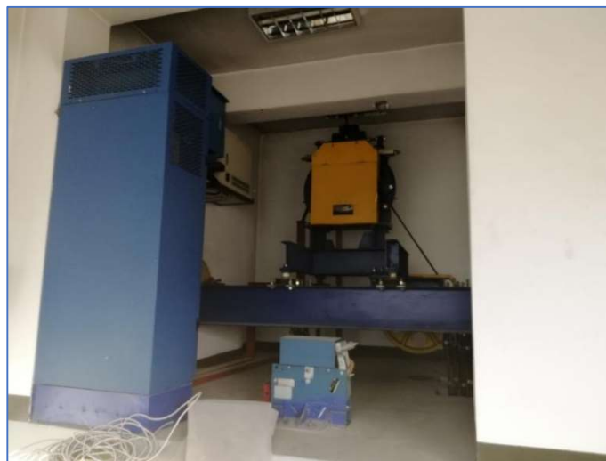
Elevator Machine Room
